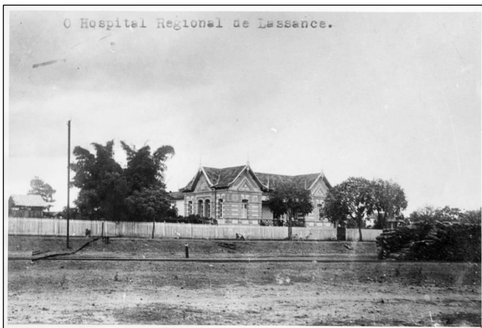
Fig.20 Hospital Regional de Lassance / Hospital Carlos Chagas Fonte: DADCOC/Fiocruz
