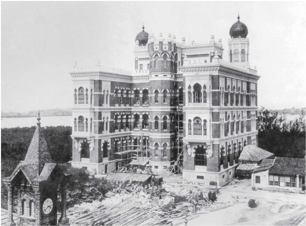
Construction of new buildings in 1908, when Adolpho Lutz was transferred to Instituto Soroterápico Federal, whose name was changed to Instituto Oswaldo Cruz in March that same year (DAD/Fiocruz).
