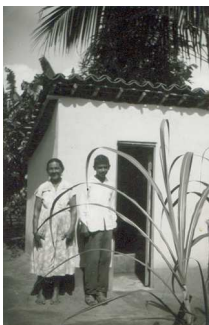
FIGURE 3- Photo “Cesspit built in cooperation with the service under the guidance of members of the Varjão Group, October 20, 1956”.
